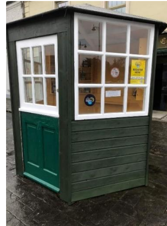
(M3) Kiosk renovation by Men's Shed
