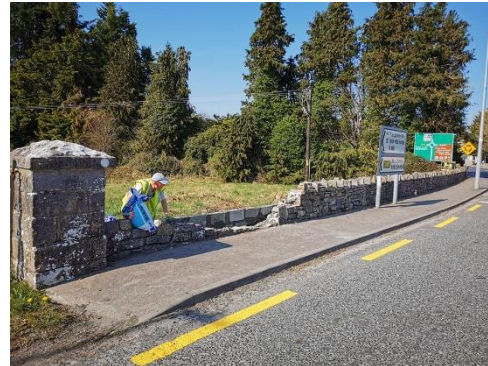
(N25) Bridge Street maintenance
